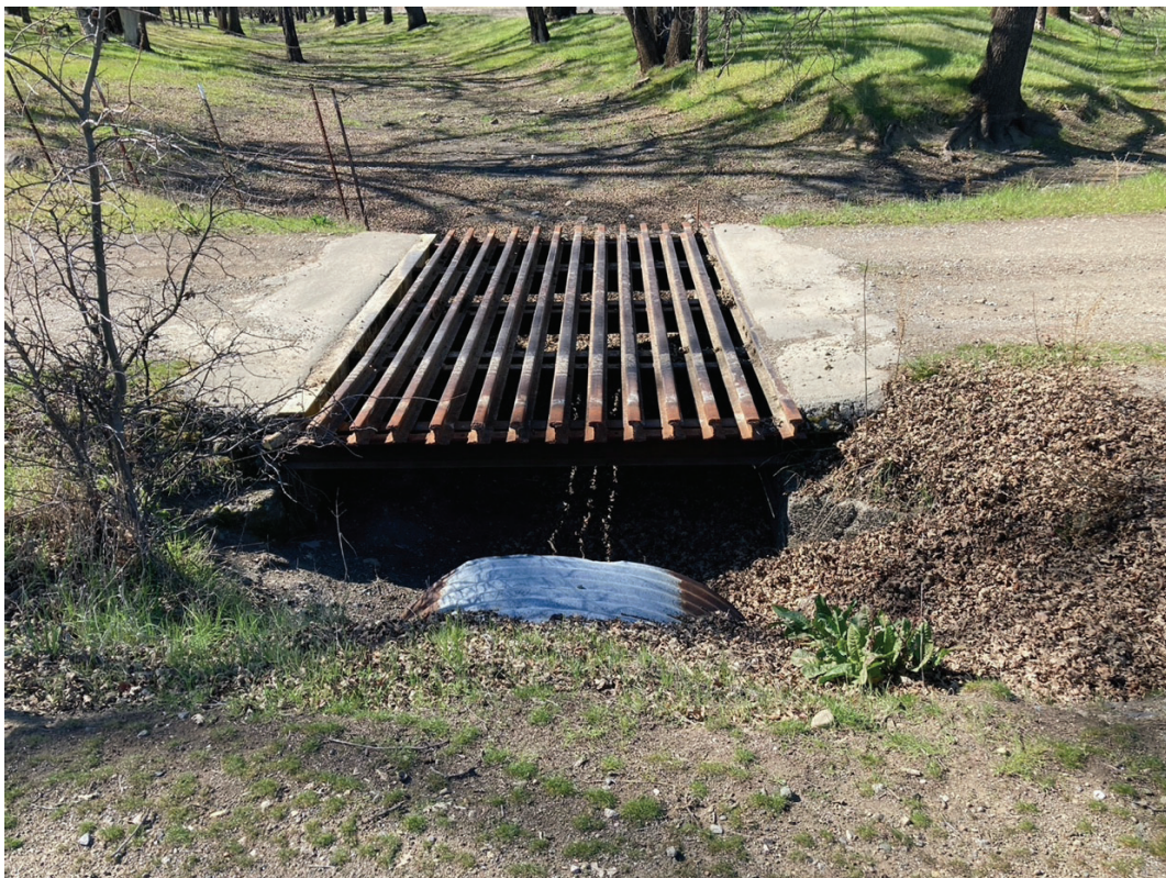
Ephemeral Class II Watercourse Crossing of Comstock Ranch Road – 5' CMP Culvert and 8' Cattle Guard
