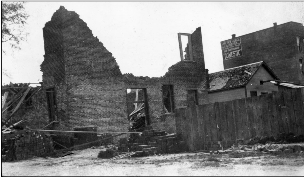
Figure 7: Possible 1906 Earthquake Damage (Lakeport)
