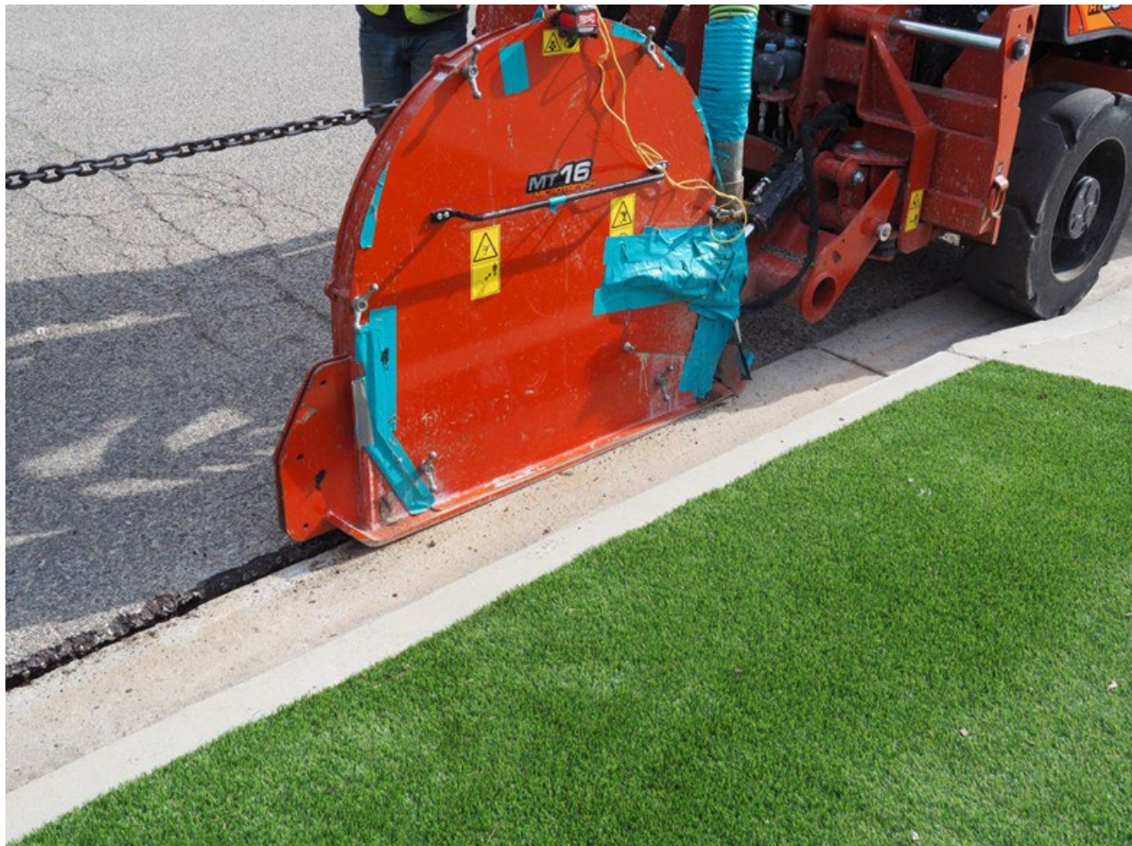
Figure B-1. The Picture Shows the Saw that Creates the “Micro Trench”. This Trench is Approximately 2” Wide and 18” Deep. An Industrial Vacuum Truck Collects the Refuse as the Cut is Created.
