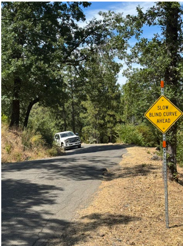
Figure 6-2 – Blind curve with limited sight distance.
