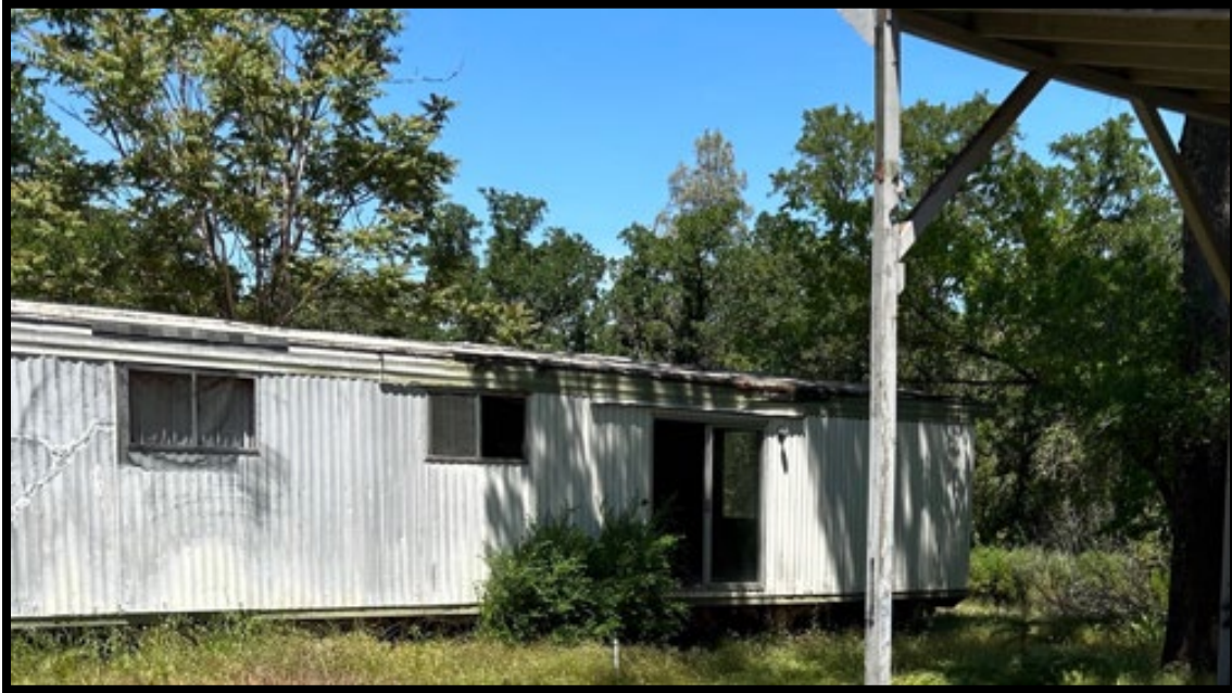
FIGURE 7 – SECOND TRAILER FOR DEMOLITION
