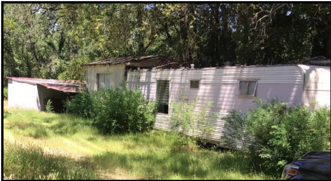
FIGURE 6 – FIRST TRAILER FOR DEMOLITION
