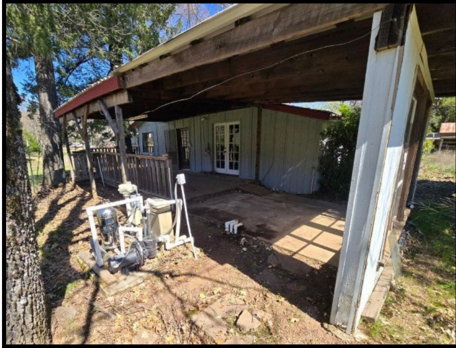
FIGURE 5 – HOT TUB REMOVAL AND CAPPING OFF OF ELECTRICAL WIRING/PLUMBING
