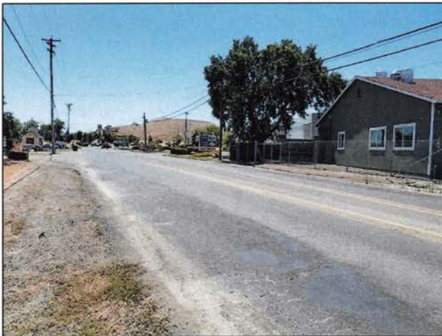
Looking south along S. Main St.
