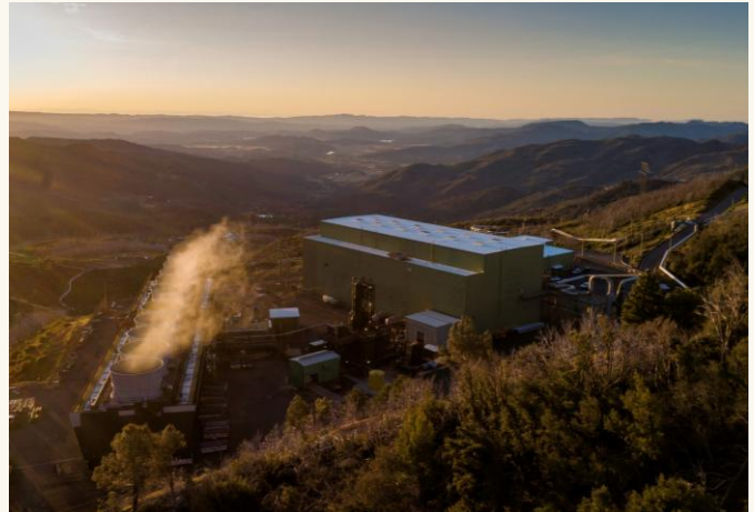
The Geysers Geothermal Power Plant generates enough electricity to power 750,000 homes.
