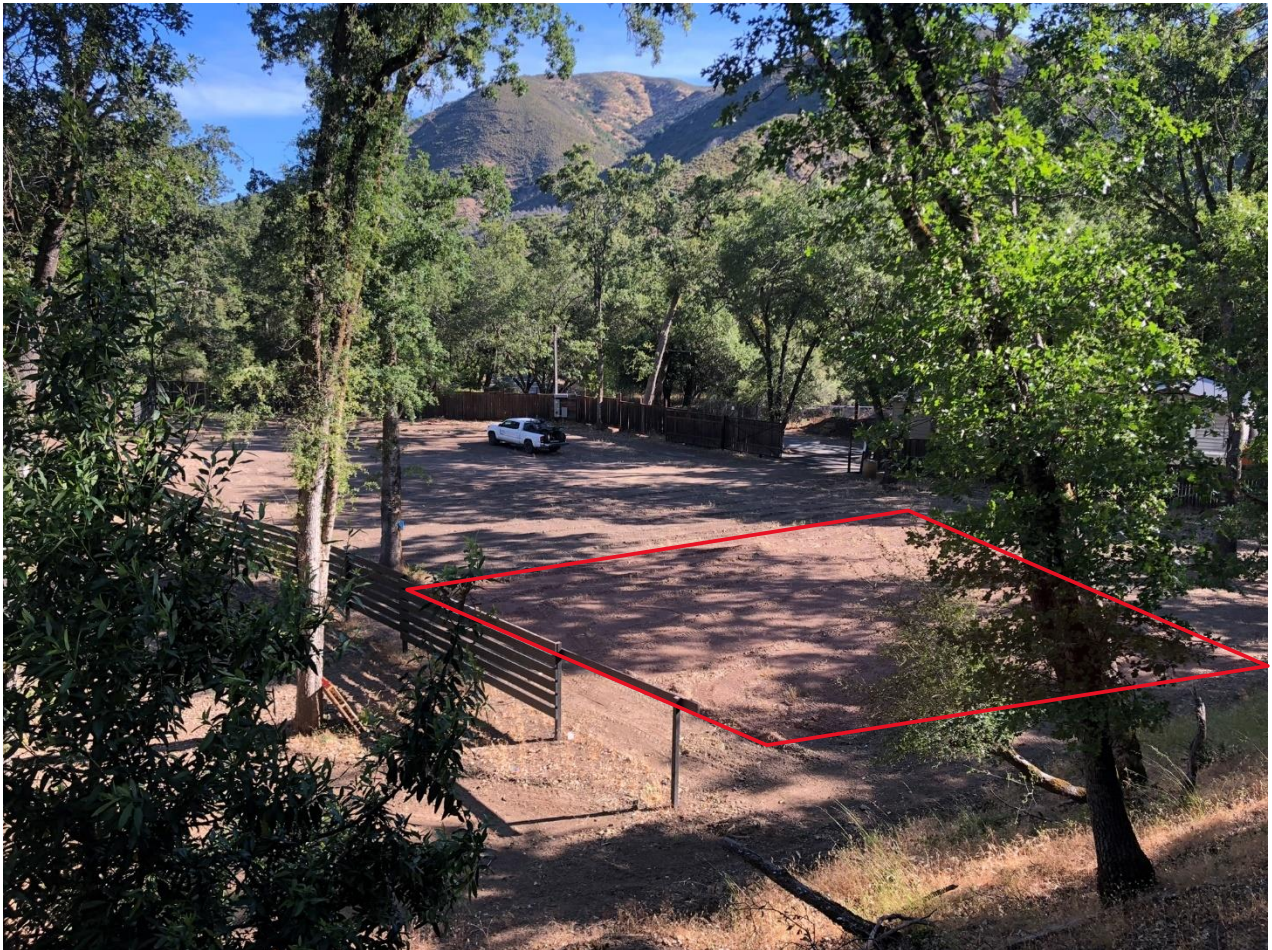
Photo 1. Looking north, this photo shows the parking lot, as well as the septic system and associated leech field site on the southern end (boxed in red). Photo taken on June 17 th by Laura Moreno-Baker.
