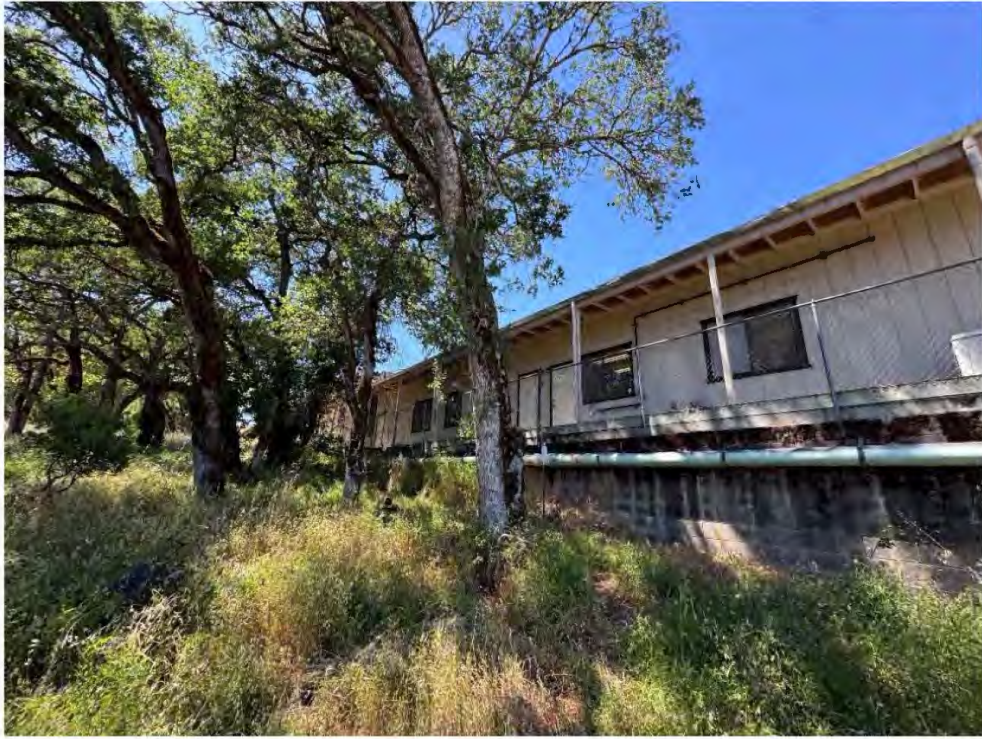
Site Photograph 9 – Looking north away from the proposed Site, May 15, 2025
