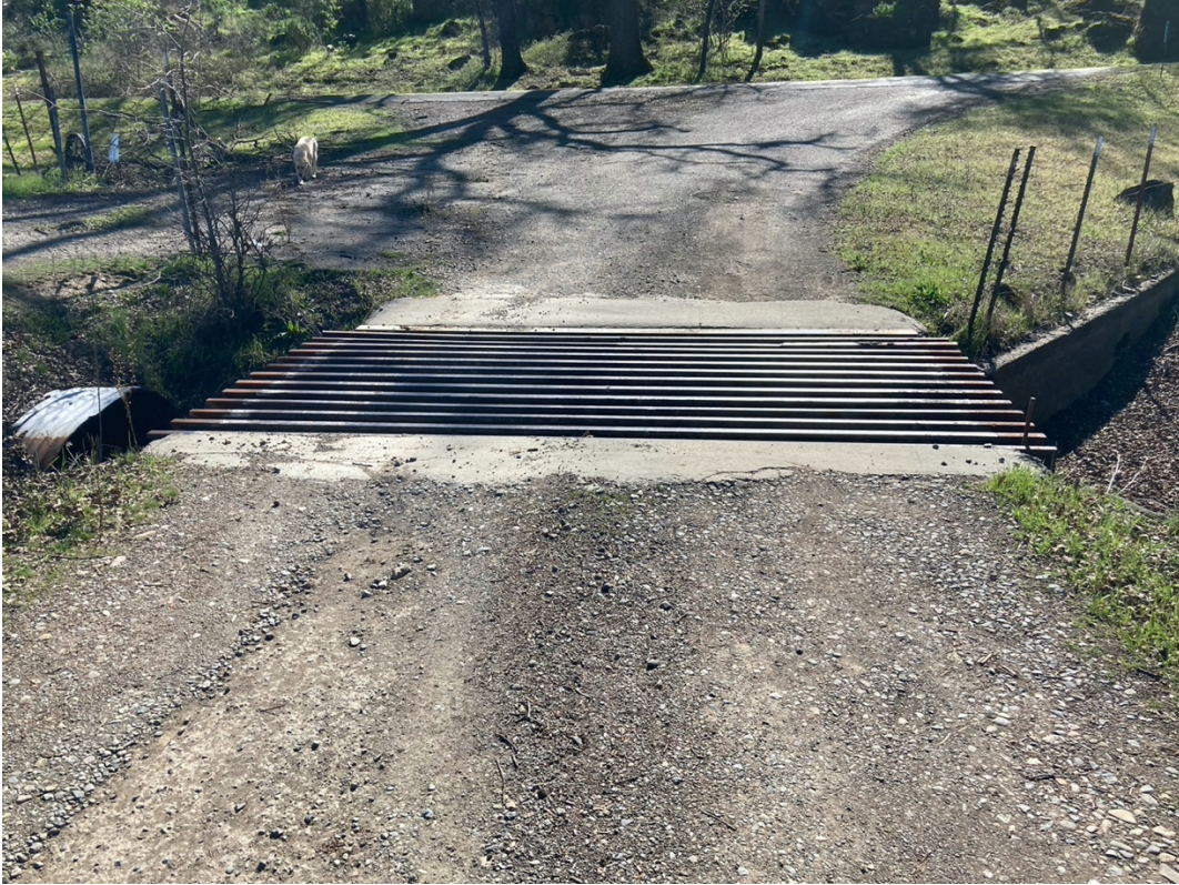
Junction of Grange & Comstock Ranch Roads (upper photo) and Class II Watercourse Crossing
