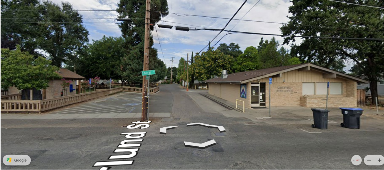
Photo of existing building, taken from Main Street
