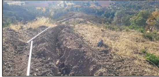
Photograph 4. Overview of waterline trench.
