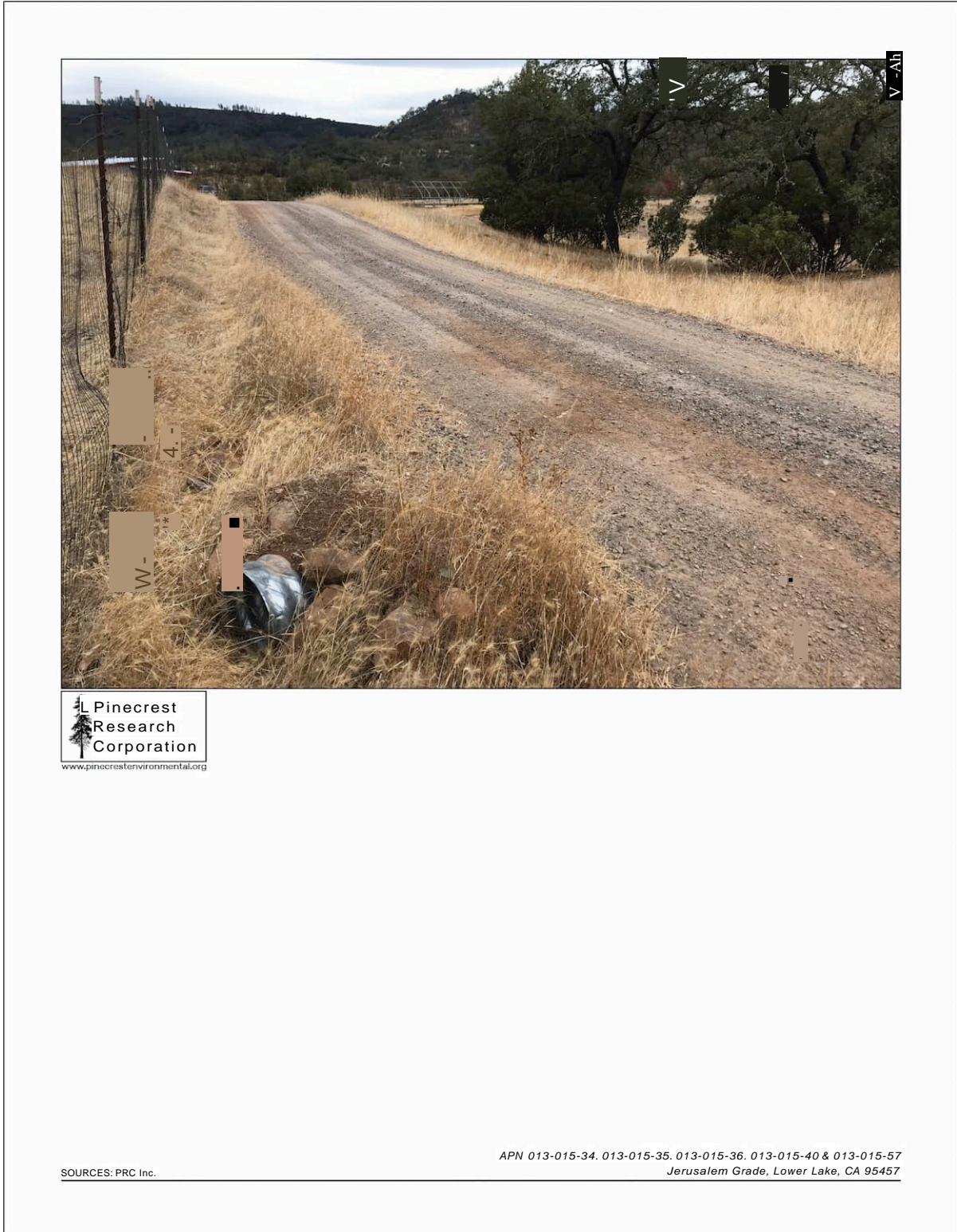
FIGURE 13: PHOTOGRAPH OF SOUTH CULVERT
