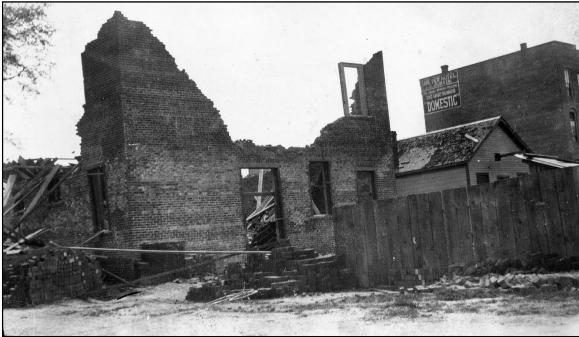
Figure 7: Possible 1906 Earthquake Damage (Lakeport)
