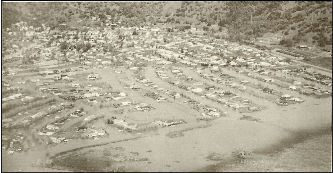
Figure 28 Historical photo of the Keys flooding in 1983.
