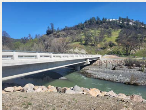
Chalk Mountain Road Bridge
