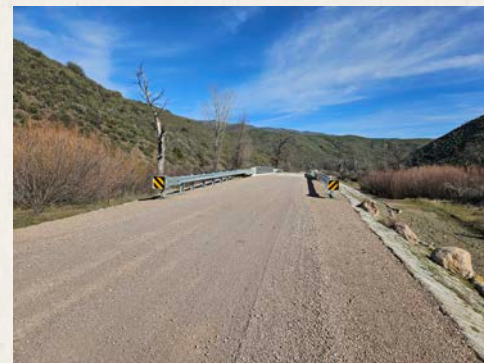
Bartlett Springs Road Bridge
