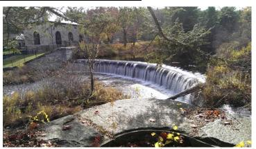
Transfer Facility at the outlet of the Quabbin Aqueduct. The dam is a 250-foot long, 18-foot high earthen embankment and stone masonry structure. The most visually compelling component of the dam is its 135-foot long 9-foot high stone masonry and concrete arched spillway. The earthen embankment portion is limited to the right side, adjacent to the granite block transfer station.
