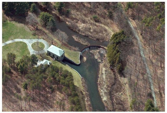
SLR was retained by the Massachusetts Division of Ecological Restoration (MA DER) to conduct an initial feasibility study and provide hydraulic modeling for the removal of the Quinapoxet Dam. The dam is a 250 foot long, 18-foot-high earthen embankment and stone masonry structure. The most visually compelling component of the dam is its 135-foot-long foot high stone masonry and concrete arched spillway.
