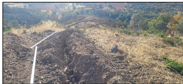
Photograph 4. Overview of waterline trench. View southeast.
