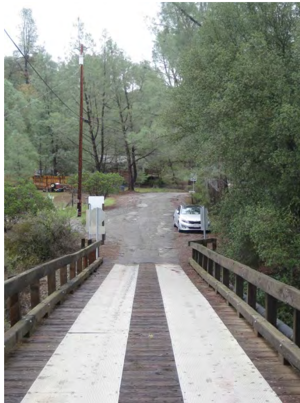
Photograph 4: Looking West- Bridge
