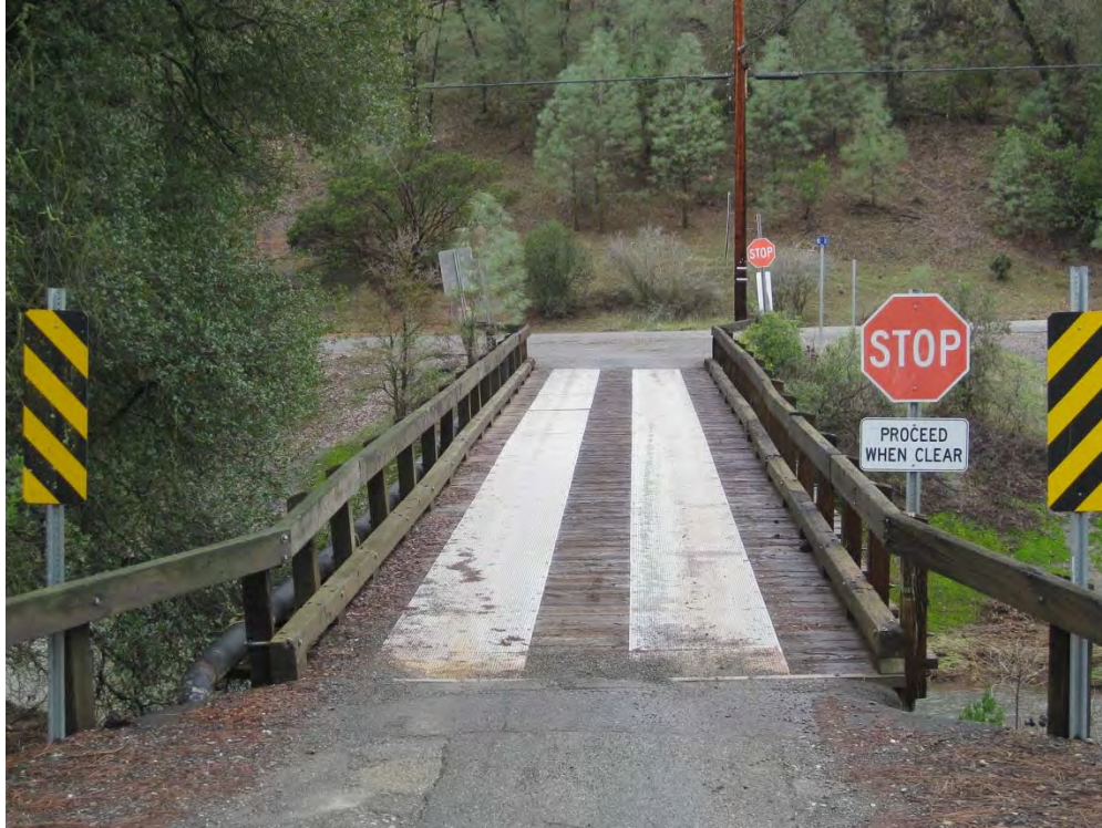
Photograph 1: Looking East- Bridge
