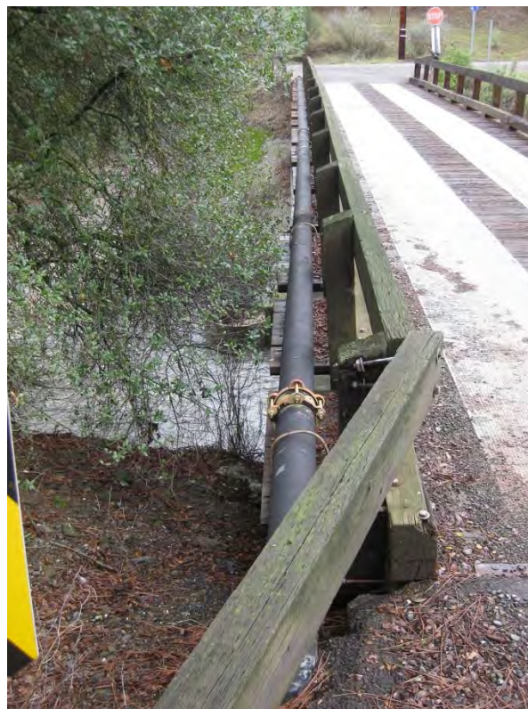
Photograph 2: Looking East- Bridge Rail and Utility
