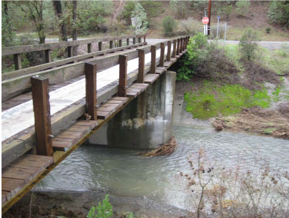
Photograph 3: Looking East- Side of Bridge
