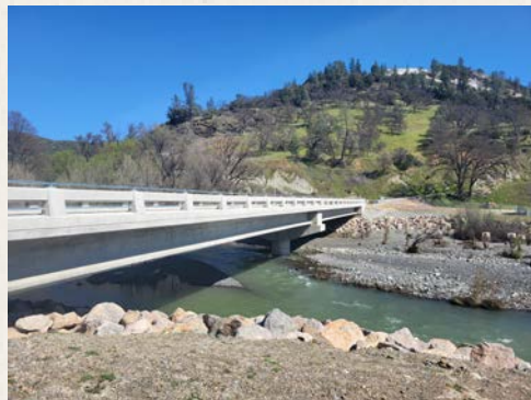
Chalk Mountain Road Bridge
