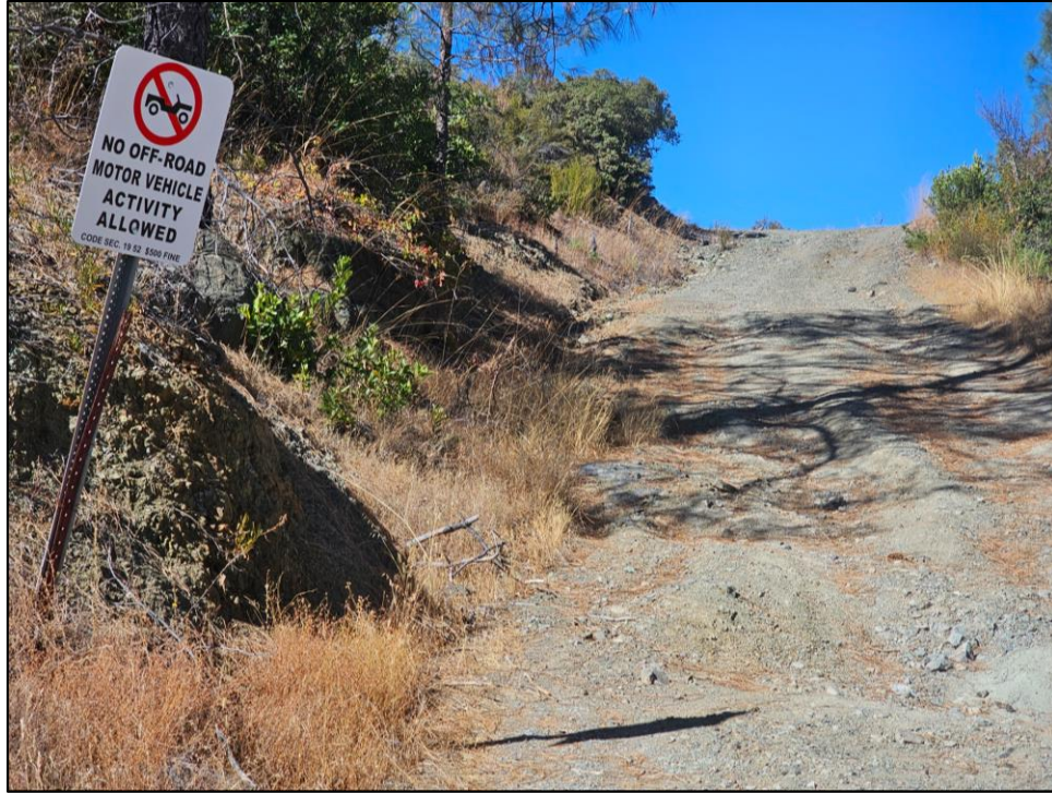
Figure A7: Ruts, steep slope and warning sign at the access road entrance
