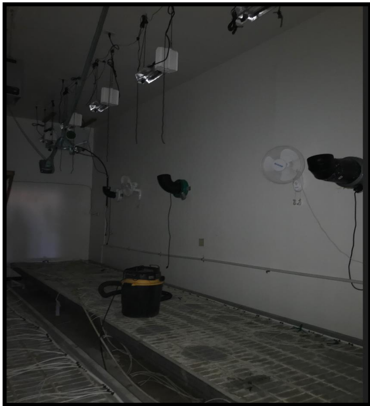
Figure 12. Grow beds, grow lights, oscillating fans, and irrigation systems in second structure
