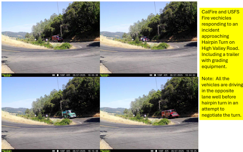
Figure E5a: Photos taken on June 7, 2025 of Fire vehicles – including trailer with bulldozer -- approaching non-compliant hairpin turn by driving in the opposite lane.
