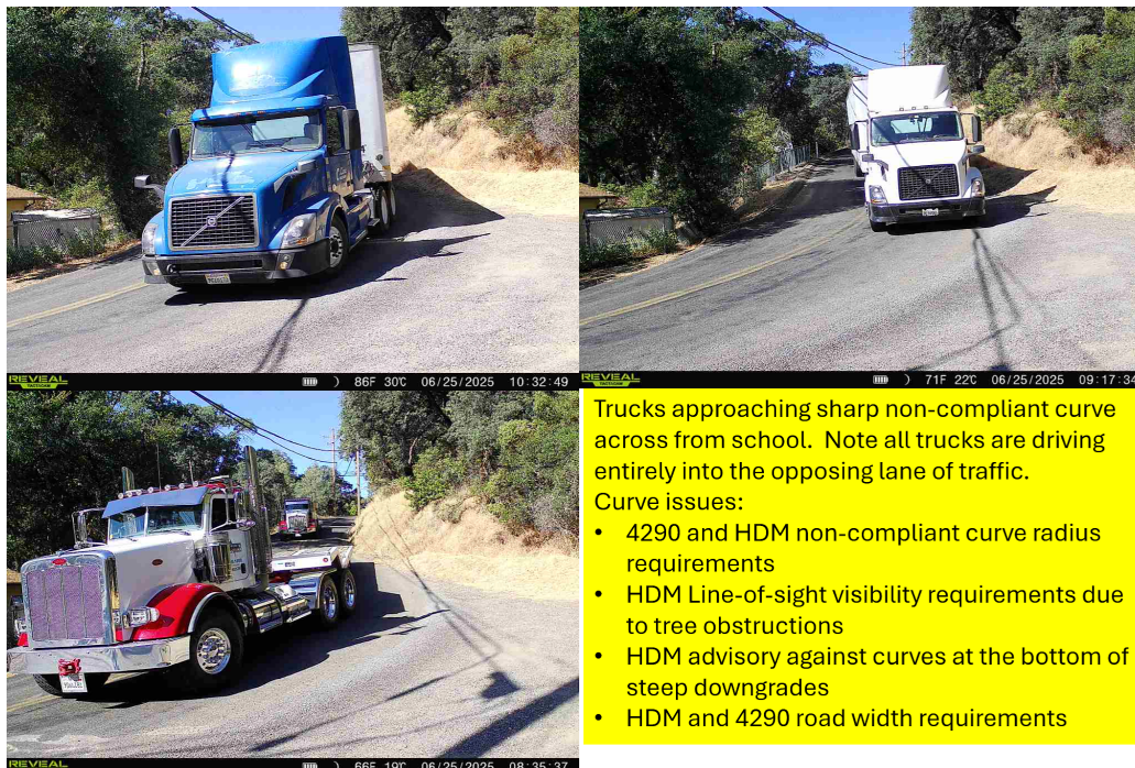
Figure E5c: Photos of Trucks driving in opposing lane of traffic trying to negotiate non-compliant curve across from the school.
