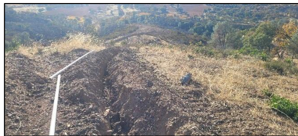
Photograph 4. Overview of waterline trench. View southeast.
