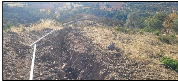
Photograph 4. Overview of waterline trench. View southeast.
