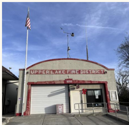
Northshore Fire Protection District operates 3 stations in the Planning Area.
