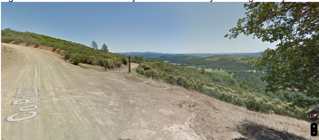
Figure 9: Eastbound View of Project Site at driveway off of High Valley Road
