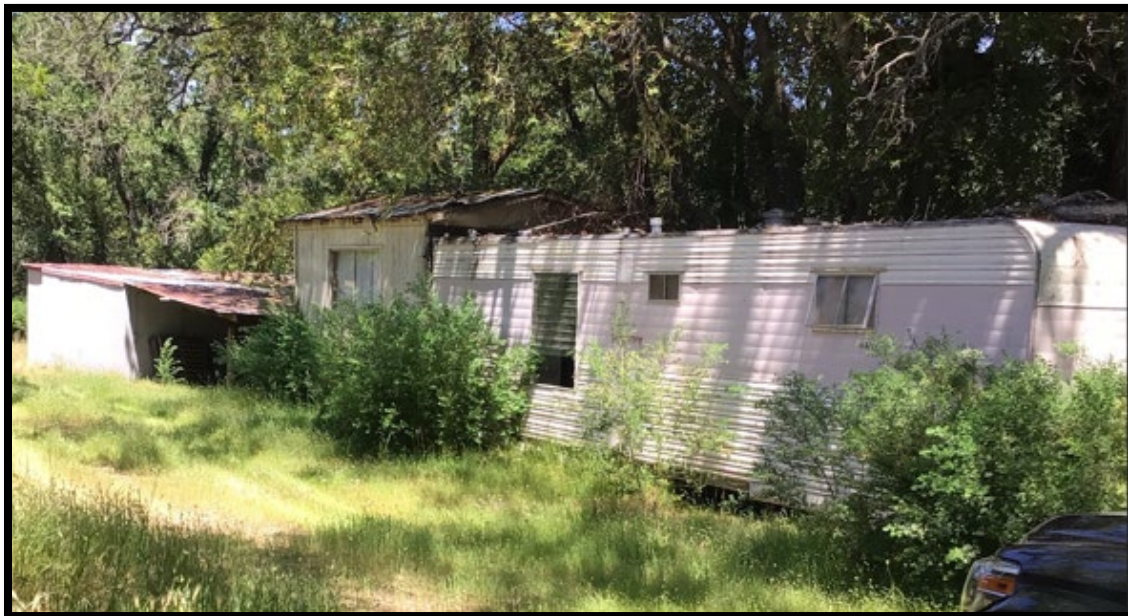
FIGURE 6 – FIRST TRAILER FOR DEMOLITION
