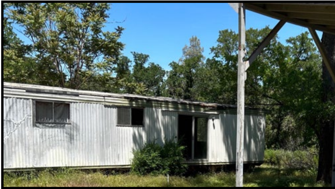
FIGURE 7 – SECOND TRAILER FOR DEMOLITION
