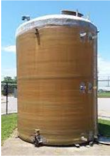
Fiberglass Water Tank
