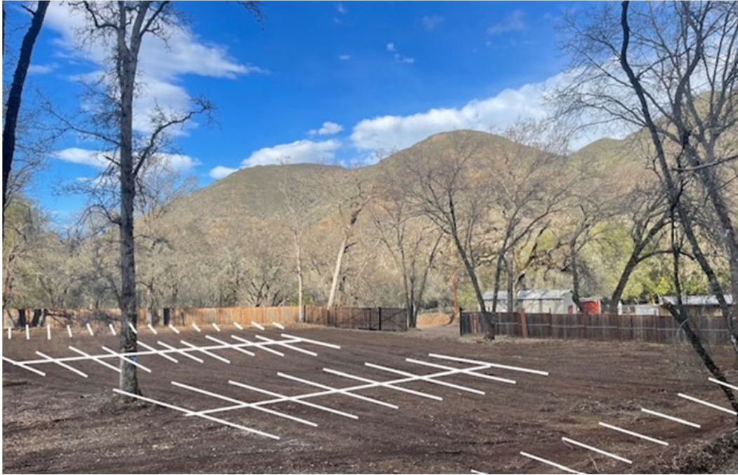
FIGURE 6 – PARKING LOT LAYOUT USING PVC PIPING AS A MOCK-UP (not to scale)
