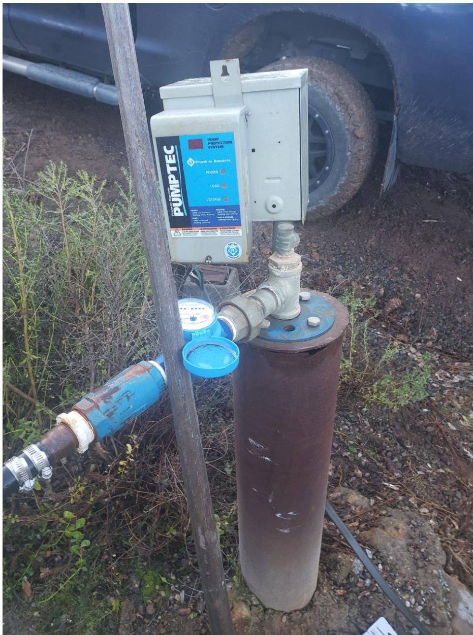
Photo 2: Close-up view of site well # 824915 and water flow meter installed at well head.
