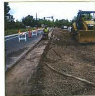
The project improved the overall transportation efficiency and **pedestrian/bicycle safety** through the construction of continuous dual left-turn lanes, an on-street exclusive bike lane, a **pedestrian sidewalk**, street parking, and landscaping. The new roadway section included the FDR process. Traffic signals at Buena Vista Avenue and Pleasant Hill Road were modified, and street lighting was improved as well.
