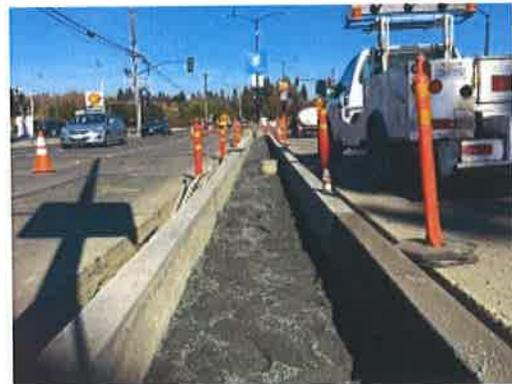
The project included the demolition of concrete curb, sidewalk, and median; excavation and grading; **new concrete curb, sidewalk, and curb ramps**; concrete pavers in the median; HMA pavement; traffic striping; street lighting relocations; traffic signal replacement at the intersection of Ygnacio Valley Road and San Carlos Drive; signage; landscaping and irrigation.
