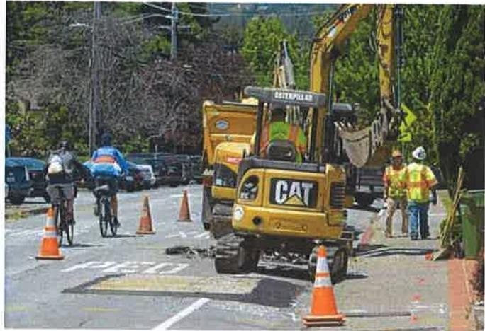
The project installs new underground utilities, recycles and rehabilitates over 8 lane-miles of asphalt pavement, **replaces sidewalks**, utility boxes, streetlights, hardscaping and landscaping to beautify over 2 miles of Miller Avenue, one of two major thoroughfares into downtown Mill Valley. Finding the right construction management team was considered crucial to the City's staff for the success of this project.
