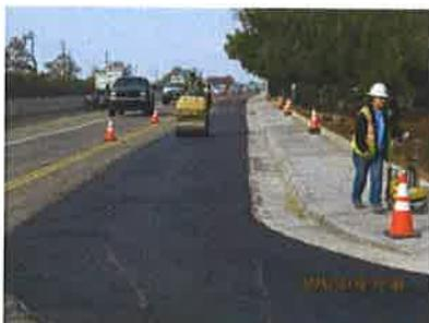
**Pavement Overlay Project:** The project installs asphalt concrete overlay along several streets throughout the City. The Project will also include the replacement of curb ramps necessary to meet current ADA requirements.
