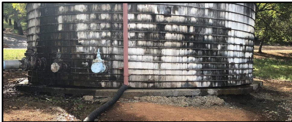
Figure 3 – Zone 1 Tank Erosion
