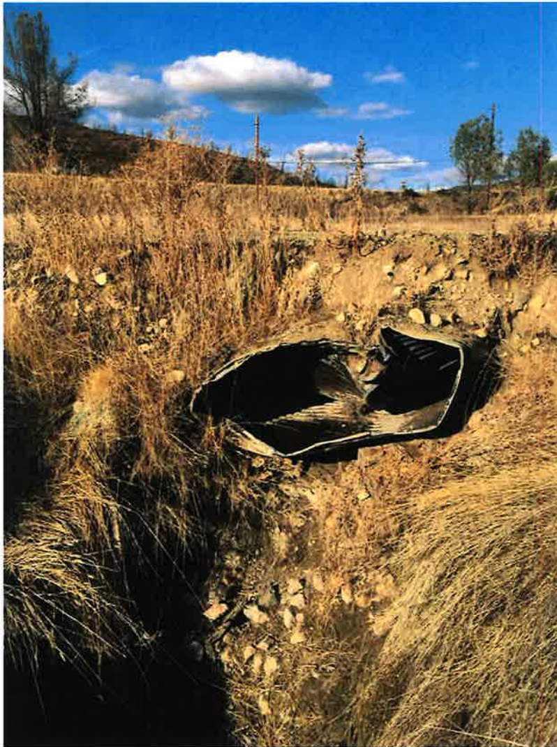
One of several broken culverts on the property that have not been replaced. The golf project will permit making much needed improvements
