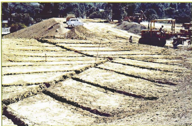
Figure 2 – Lateral lines should be spaced not more than 15 feet (5m) apart and have a natural fall to the mainline of at least 0.5%.
