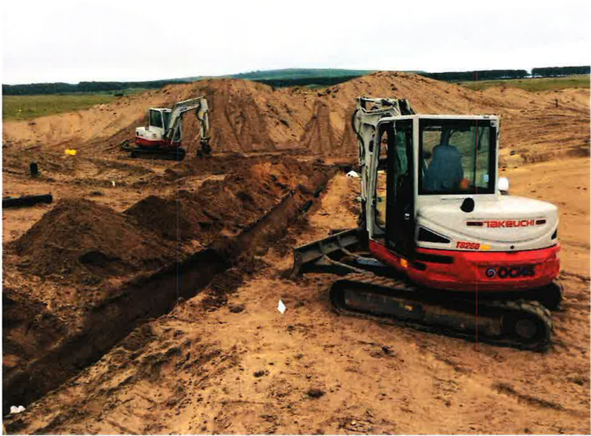
Example of golf course drainage construction. Dumbarnie Links, currently under construction.
